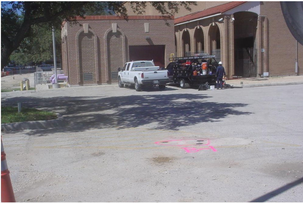
Photo 1 – View looking towards the northwest at the attempted locations of Boring B-1.
